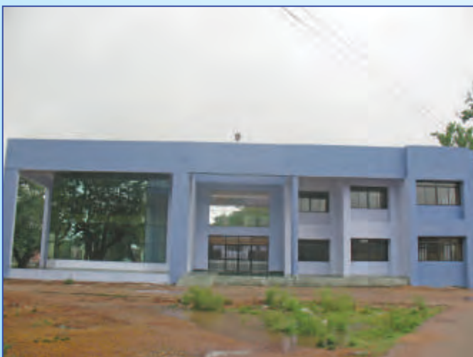
New Administrative Building of ETC, Hehal
