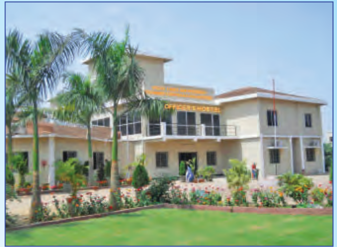
Hostel of Watershed Training Center, Nagri
